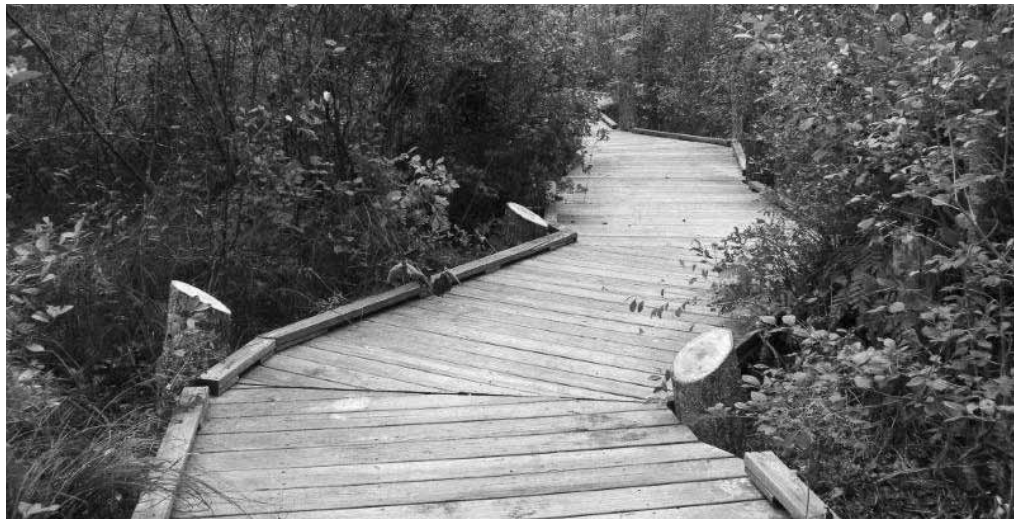
The boardwalk to the lake through wetlands at Constitution Park received new footings and other improvements this year thanks to a grant obtained by the Town of Ossipee. Photo: Jean Hansen
