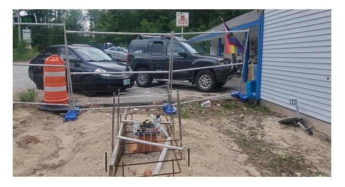
The picture shows the form work and rebar for the Diesel Pump concrete pad. In the middle is the piping and electrical conduit, which will extend up out of the concrete to be connected to the pump. Behind it are the residential apartments, residents' cars and their parking spaces.
